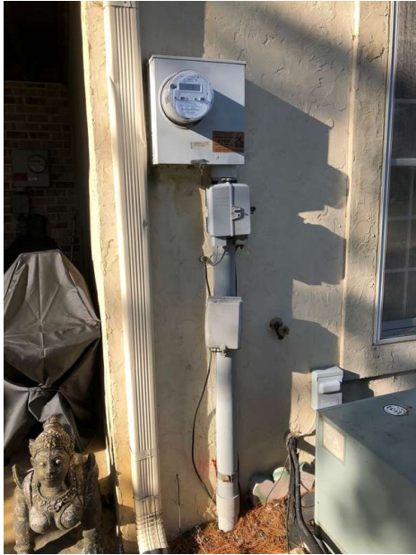
Typical Underground Service
