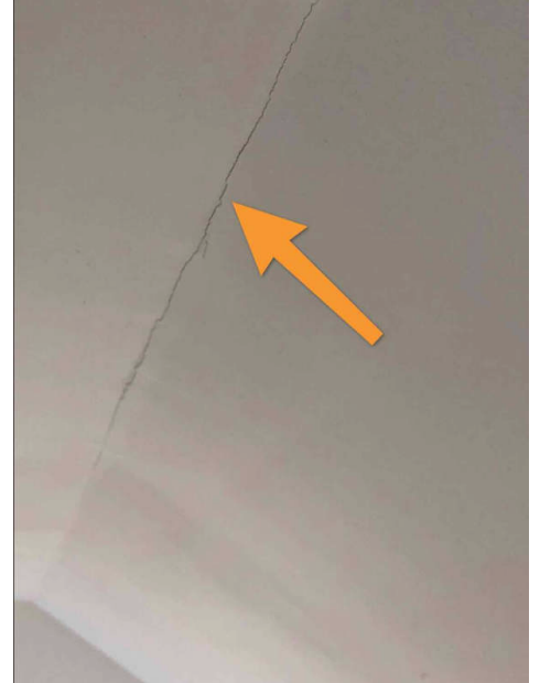
cathedral ceiling dining room
