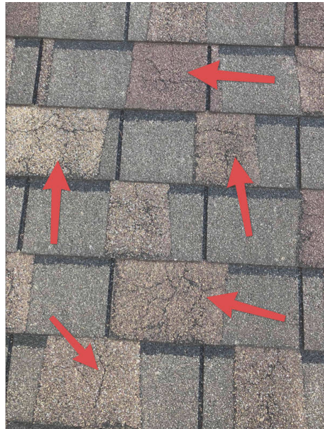
cracking shingles
